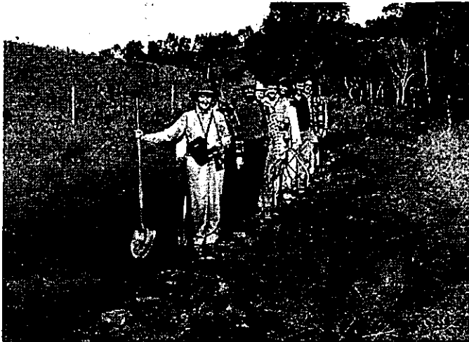
Budawangs. Placing stepping blocks (cheeses) in a muddy section of the track, one of several work parties in the Budawangs between the Wog Wog trackhead and Bibbenluke. Other work involved track construction, re-routing, stabilisation and maintenance.
