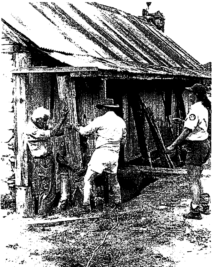
Orroral Homestead. Replacing a corner post from the rear verandah.
